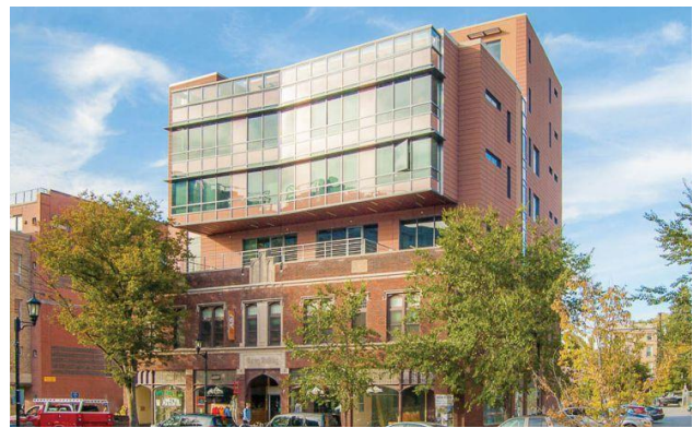
Figure 12: Carey Building (Credit: Travis Hyde)
