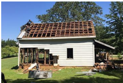
Photo by Demolition Deconstruction
